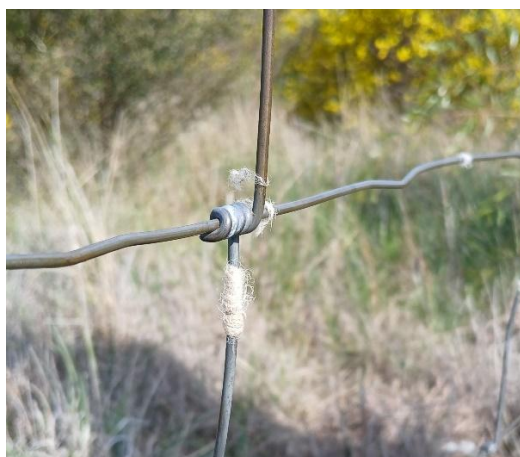
Figure 3. Hinged joint fencing has a tightly wrapped knot which is flexible enough to withstand moderate stock pressure. It is recommended a 'hot' wire be installed if cattle or horses are present.
